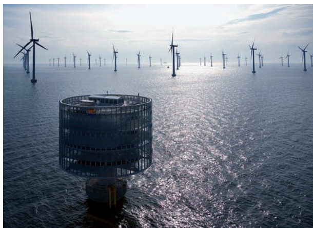
FIGURE 2 An offshore wind farm between Malmö, Sweden, and Copenhagen, Denmark, that delivers a power output comparable to that of a large coal-fired power plant.
